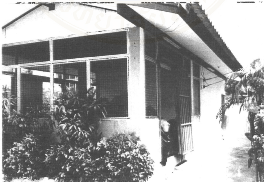
Figure 7 Normal Waste Disposed in storage room in Pranangklaao Hospital
