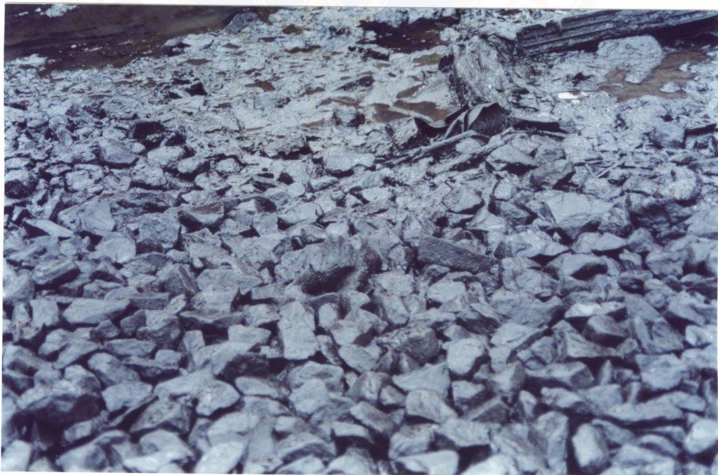
Fig. 3-2 The contaminated gravel at Band Sue Diesel Locomotive Depot
