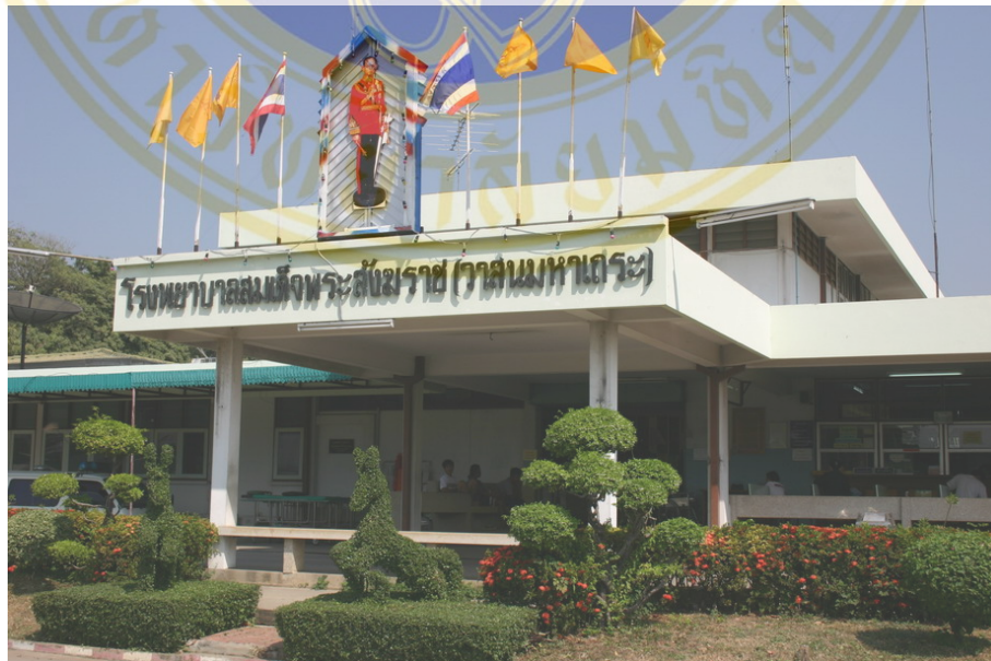
Figure 4.2 A photograph of OPD building number 3130/2526
