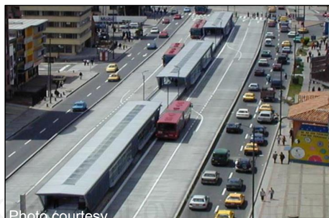
Figure 3.7 The multiple stopping bays (platforms) in Bogota's BRT
