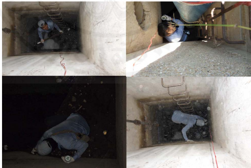
Figure 3.7 Spot measurement of flow and depth
