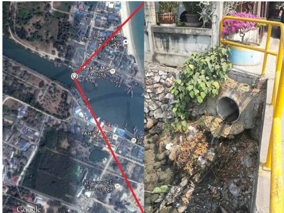
Figure 2.4 Combined sewer pipe flow to the canal
