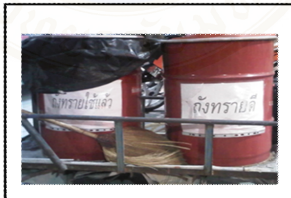
Figure 4.46 Absorbent was provided to protect chemical spills or leaks
