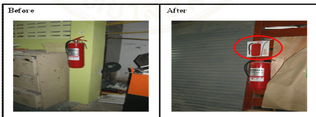
Figure 4.31 A sign showing a location of portable fire extinguisher is marked in printing factory B
