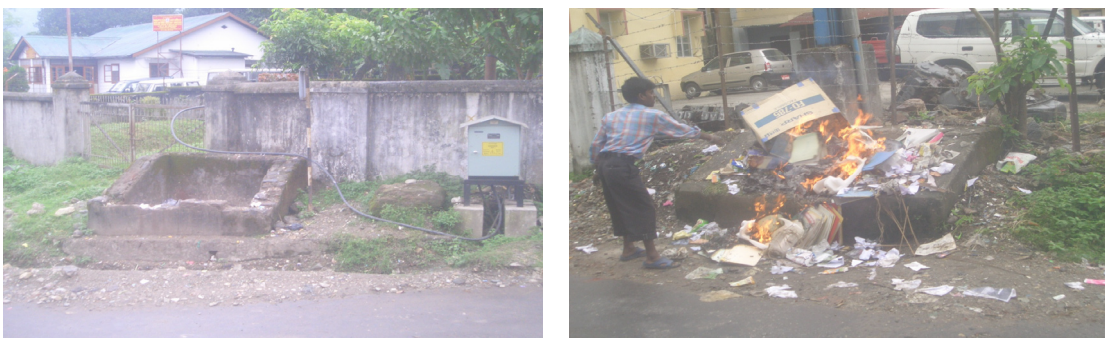
Figure 4.4 Existing conditions of concrete bins in Phuntsholing city in 2007
